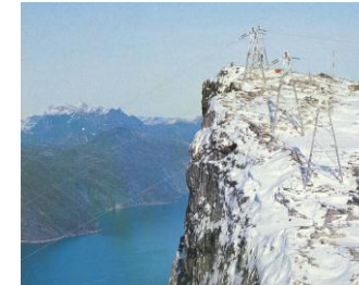
Figure 1 - Fjord Crossing Greenland - TB 396
